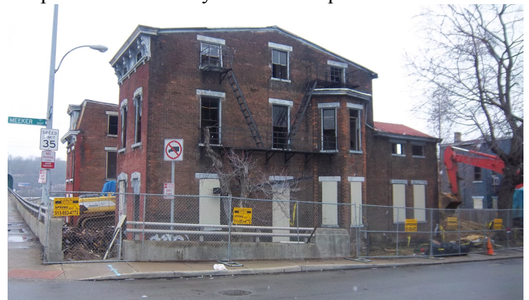
Three vacant houses are torn down at Hopple at Meeker.
